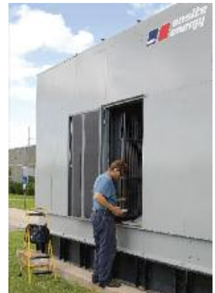
Figure 3. Regular exercise and maintenance of the complete power system are very important factors in high reliability.
