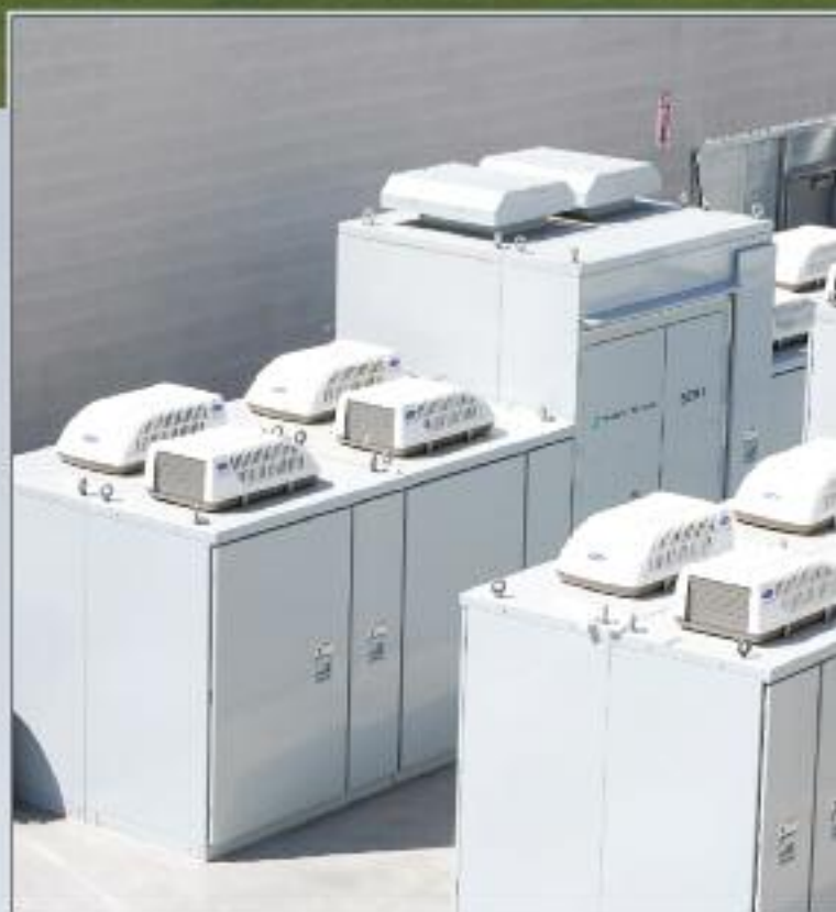
Medium-voltage PureWave UPS System
