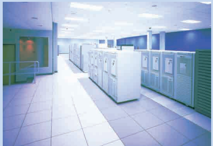
12,000-SF datacenter on a 12-inch raised floor with N+1 redundancy for cooling and electrical infrastructure.
