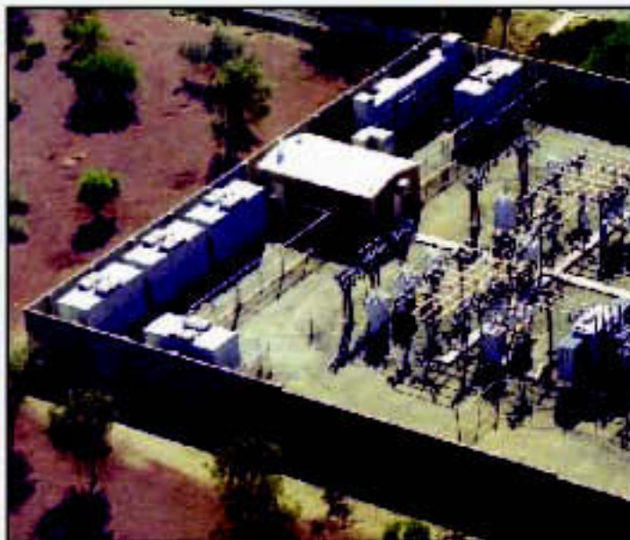
S&C PureWave UPS System rated 12,500 kW @ 12.47 kV protecting a large critical load
