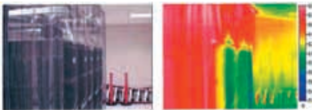
Figure 1.4 Improved Computer Room Photograph & Thermograph
