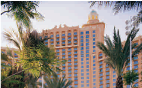
JW MARRIOTT ORLANDO GRANDE LAKES 4040 Central Florida Parkway Orlando, FL 32837
