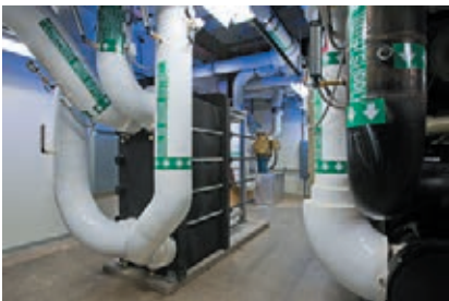
Plate and frame heat exchanger that enables chillers to be shut down to save energy and eliminates introduction of outside air to IT equipment
