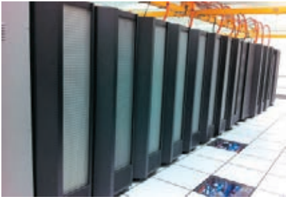
Rear door heat exchangers shown here in our Singapore Data Center have proven to be a reliable, energy efficient cost effective technology
